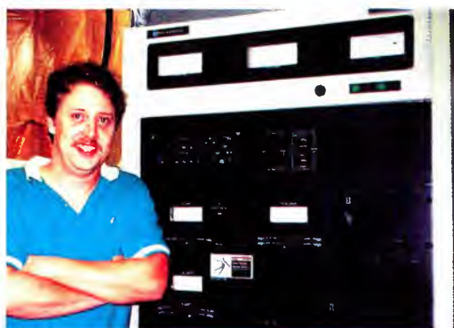
Chief Engineer Robert LaFore WITH HIS NEW HARRIS HT 20FM 20 KW FM TRANSMITTER.
